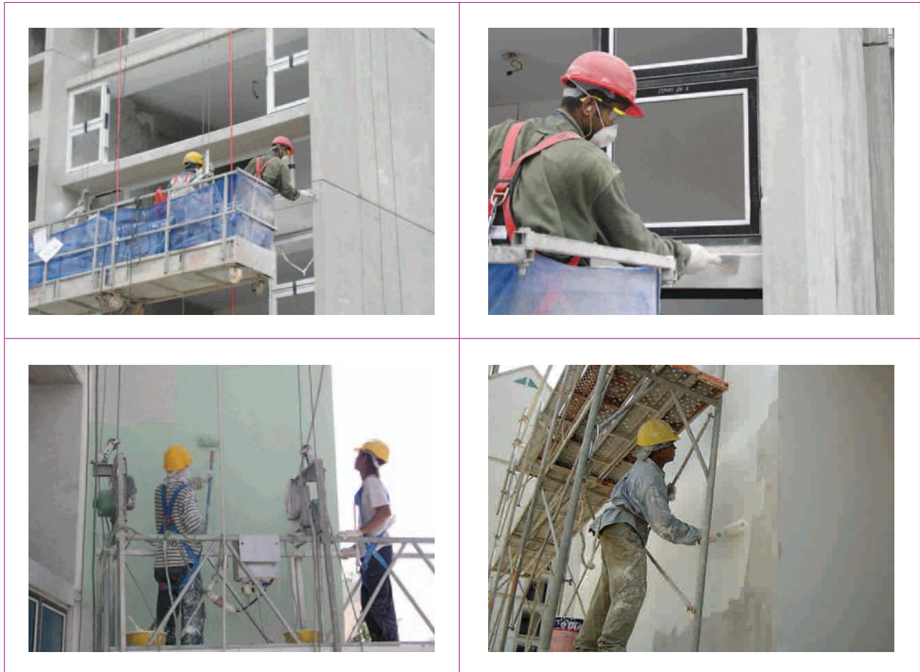
Figure 4.2 Proper access and safety measures for surface preparation and external painting works
