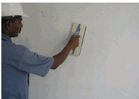
Figure 5.1 Sanding between coats of paints
