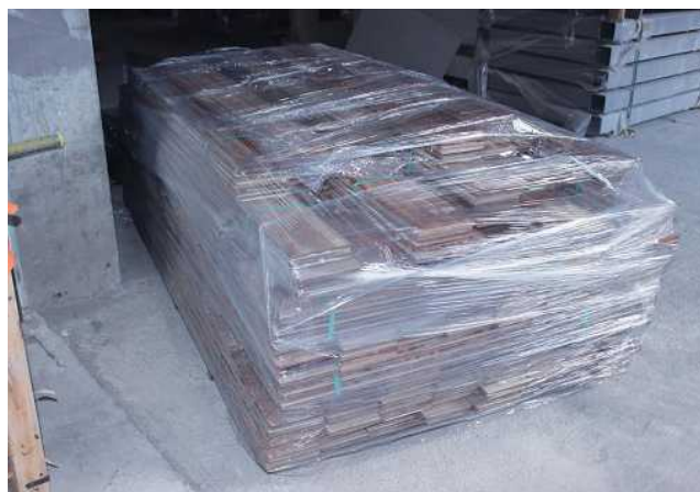
Protection intact on site before installation
