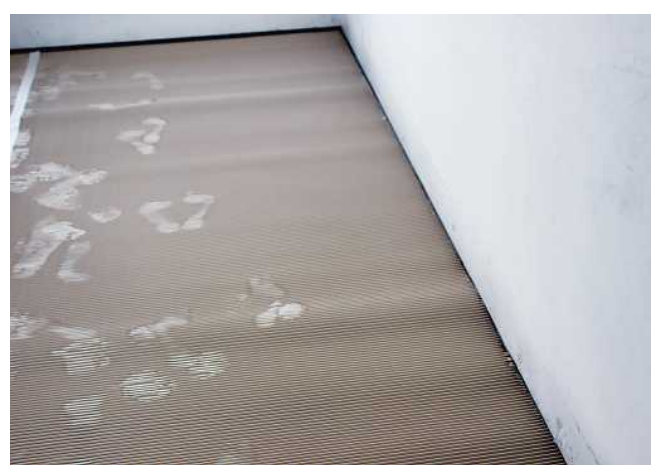
Floor finishes covered with cardboard after installation
