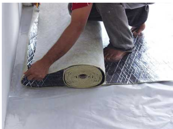
Installation of underlay material
