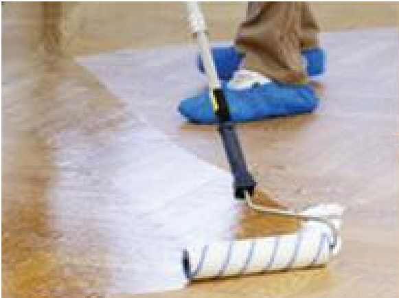
Apply protective coating
