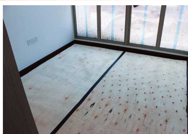
Floor finishes covered with plywood (thickness - 3mm) after installation
