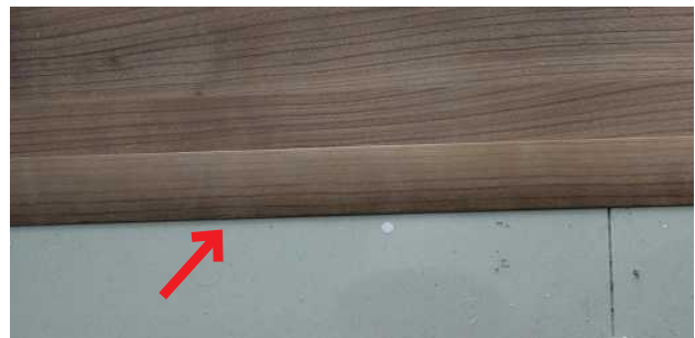
Joint with Capping
