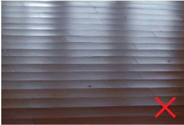
Cupping of engineered wood flooring
