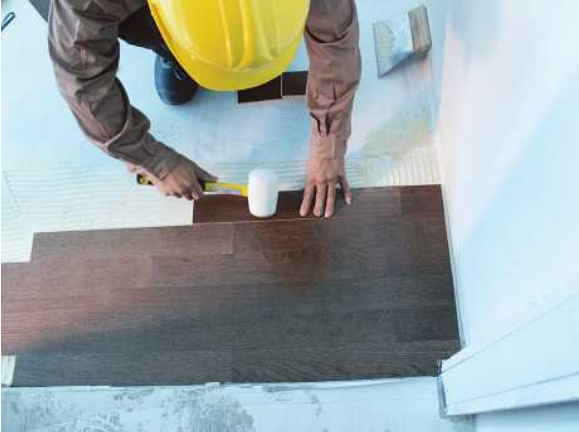
Use mallet and tapping block to install boards
