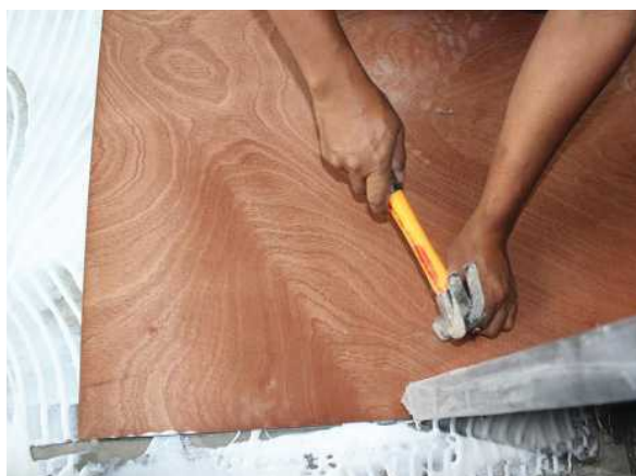
Installation of underlay material
