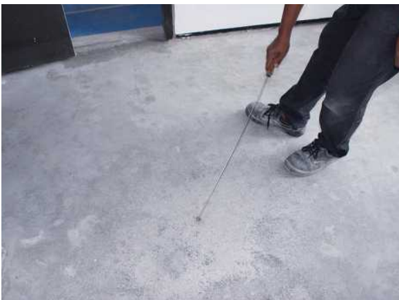
Check the soundness of the receiving floor
